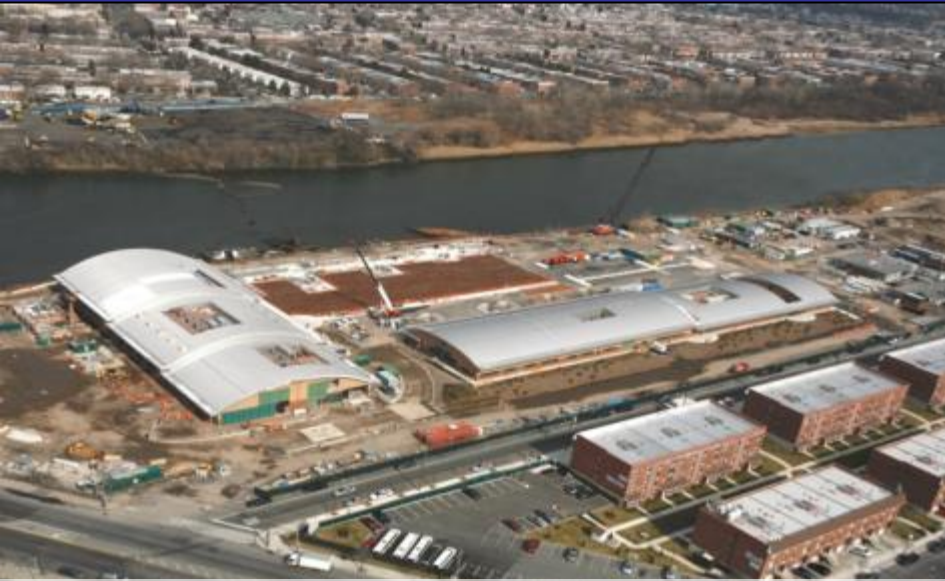
Paerdegat Detention Facility
